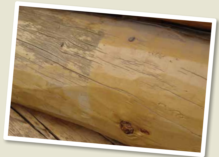
1 coat (left) vs. 2 coats (right) – it makes a difference!
