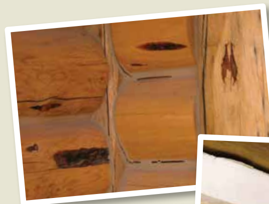
Cohesive failure of chinking
