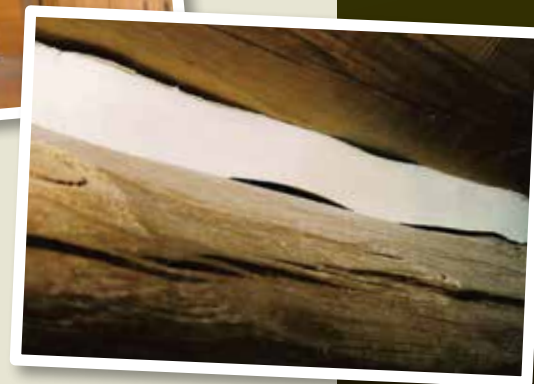
Adhesive failure of chinking
